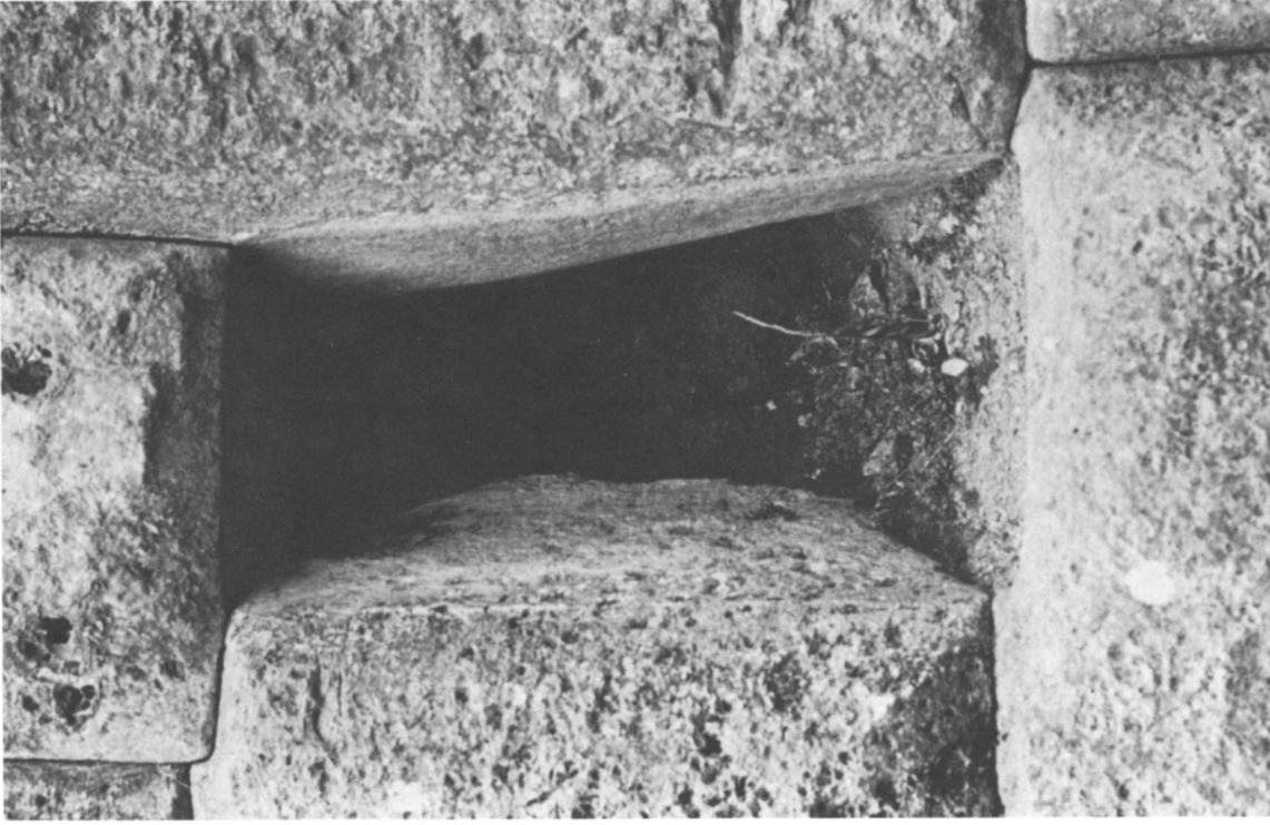
Fig. 31 , illustration of the combined effect of the fitting of bedding joints and lateral joints at Saqsawaman; fig. 32 , gap left by keystone fallen out of bond; notice taper of sides of gap, leaving a wedge-shaped hole; since hole is wider at the bottom than the top, keystone must have been introduced from the front.
