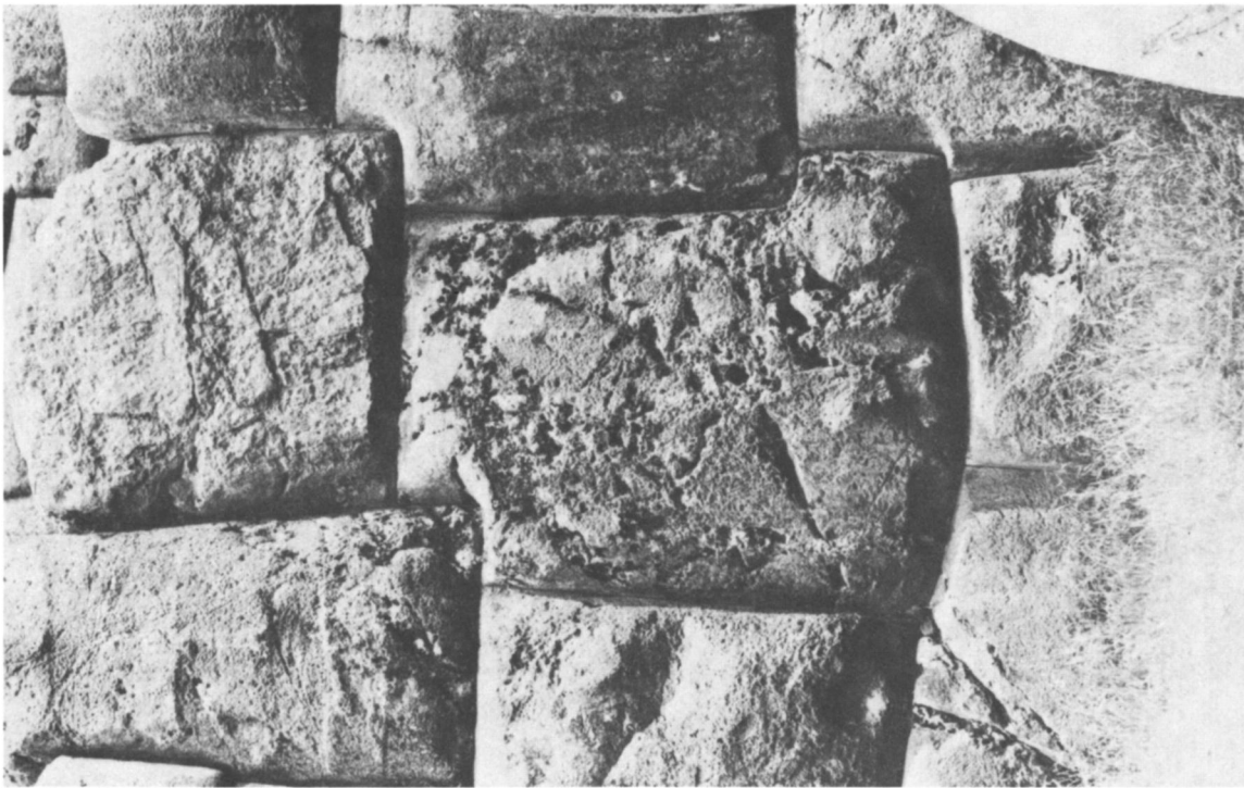
Fig. 31 , illustration of the combined effect of the fitting of bedding joints and lateral joints at Saqsawaman; fig. 32 , gap left by keystone fallen out of bond; notice taper of sides of gap, leaving a wedge-shaped hole; since hole is wider at the bottom than the top, keystone must have been introduced from the front.
